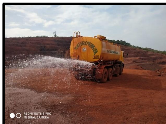
(Water Sprinkling on Haul Road)
