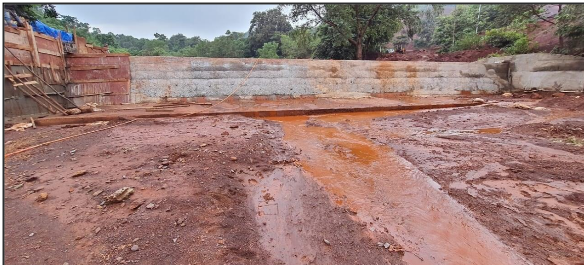
(View of check dam)
