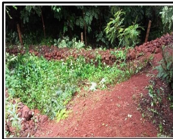
(View of Retaining wall around OB Dump)
