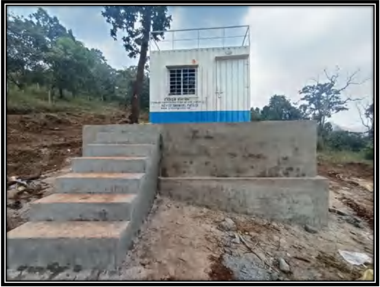
PHOTOGRAPH SHOWING INSTALLATION OF ONLINE MONITORING SYSTEM
