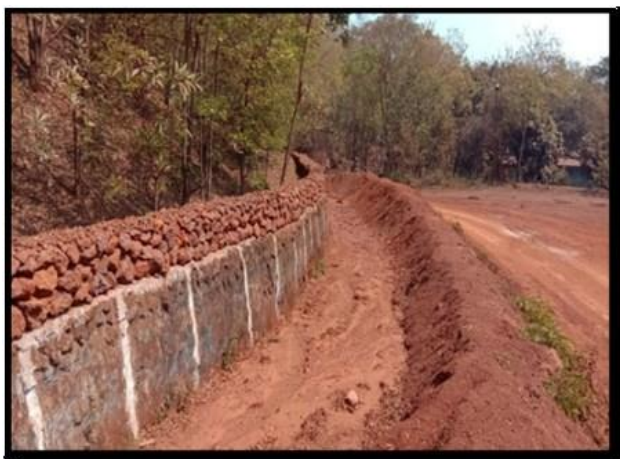
(View of Retaining wall around SG Dump)
