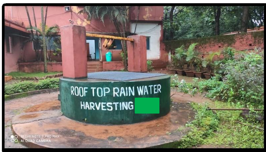
(View of Roof Top rain water harvesting str)
