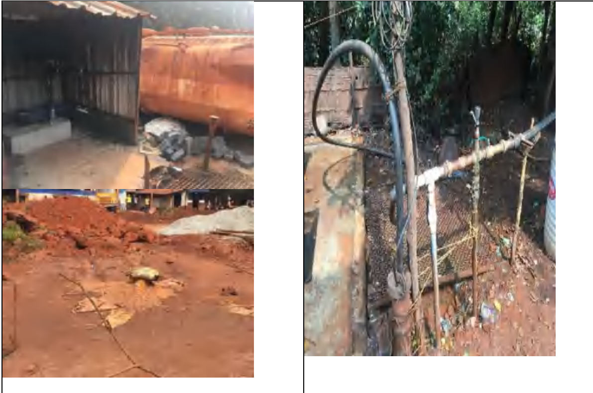
Picture 1: Photos of Bore well
